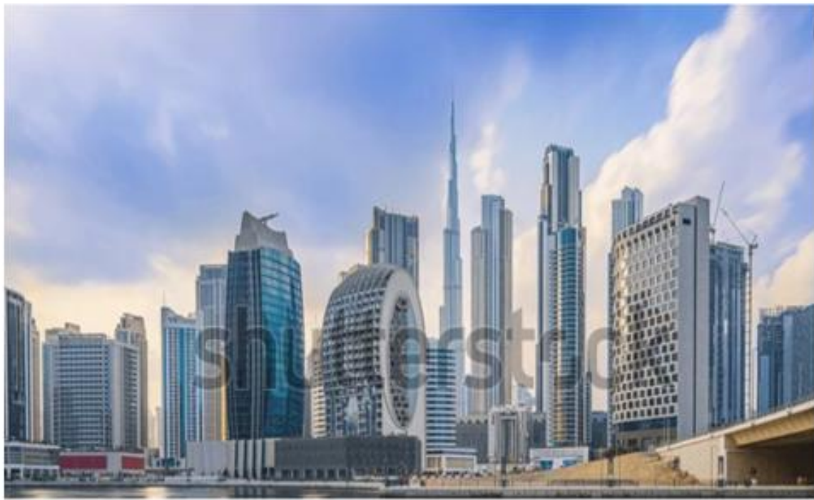
Large Building Facilities: Commercial and residential buildings needing integrated management systems, smart lighting, and security.
